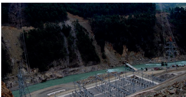
Uzundere Hydroelectric Power Plant, Turkey Learn more about the hydroelectric power plant in Turkey here.
